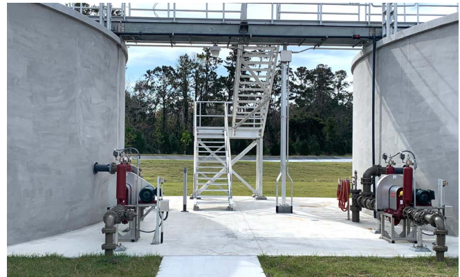
Direct pipe scum pumping installation in Florida.
